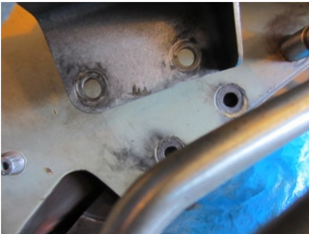
Picture 5: L/H broken front frame bolts
