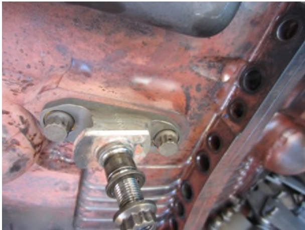
Picture 7: VSV mount bolts without safety wiring
