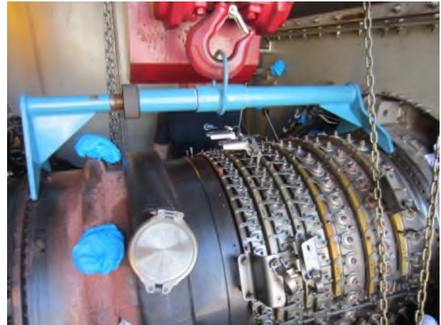
Picture 8: Top case lifter installed
