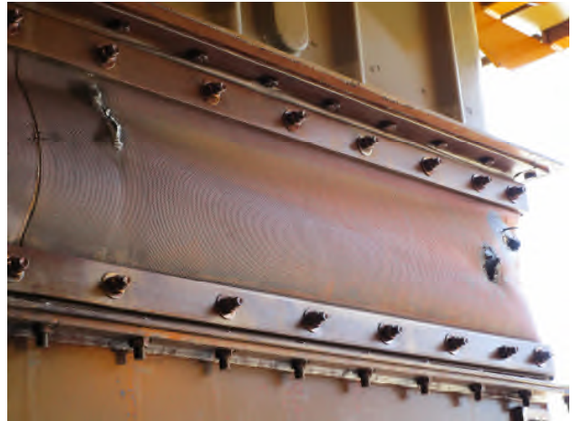
Picture 4: VBV duct bellow - damages
