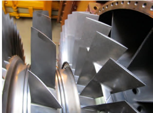
Picture 16: new installed stage 1 blade set
