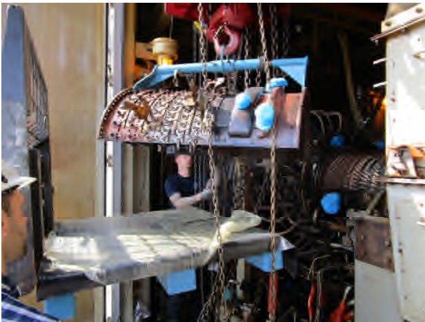
Picture 17: HPC upper case installation
