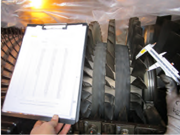
Picture 13: stage 2 - 4 blade chord measurement
