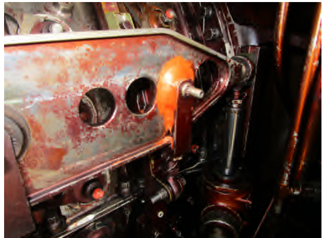
Picture 6: missing viton boot right hand side
